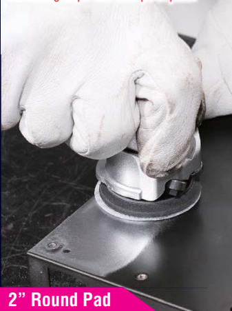
Removing drips and clumps of paint
