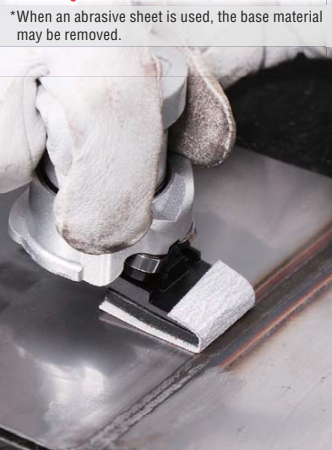
Removing weld discoloration on stainless steel
