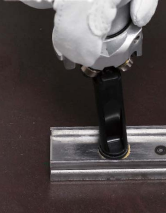
Removing the oxidized discoloration caused by spot welding
